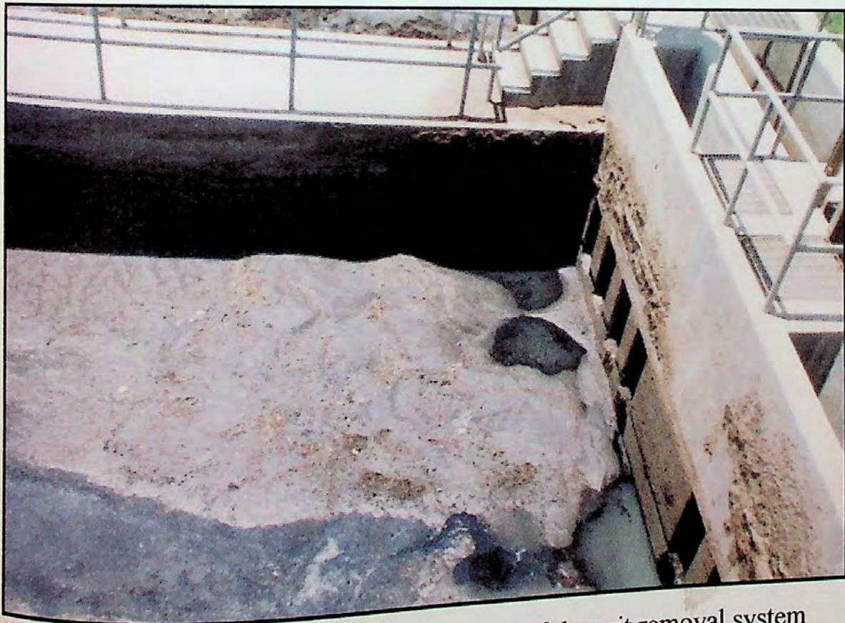
Fig. 39 : K) Dumping area of the grit removal system
