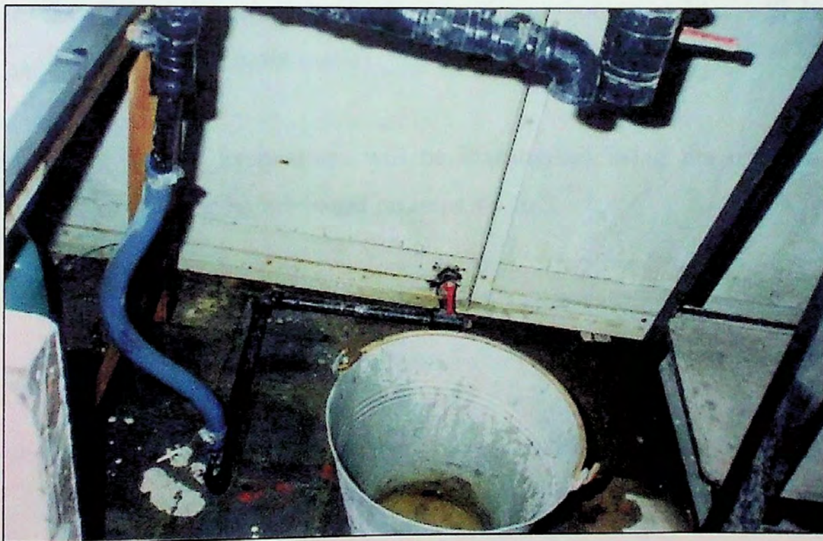
Fig. 24 : I) Tap water source connection
