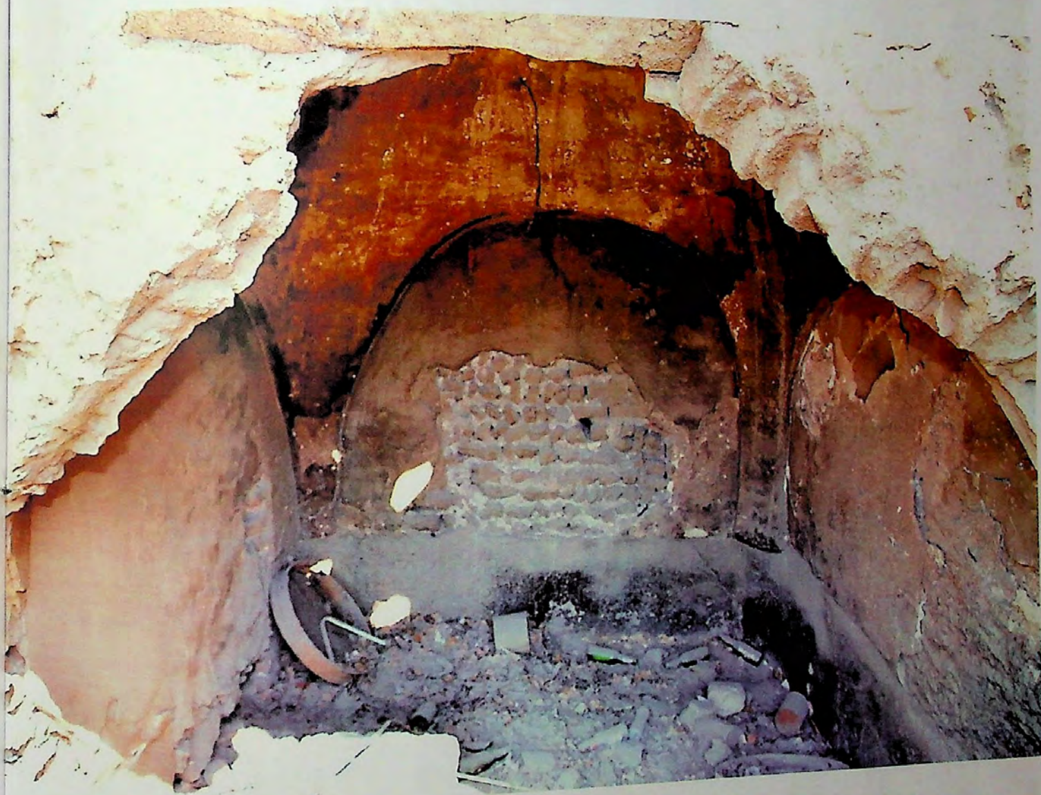
Figure 5.26. The vaulted hammam now accessible from one of the pierced recesses of the double height hall.
