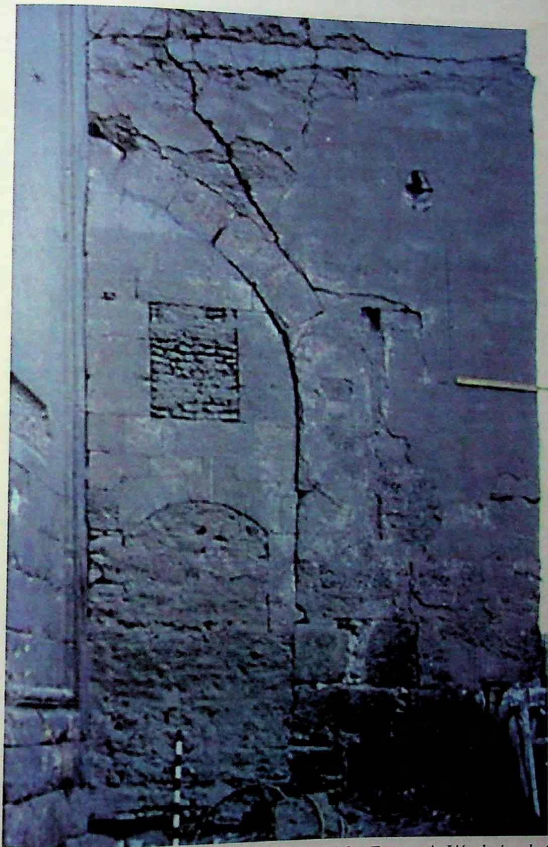
Figure 4.61. The entrance that was once right beside the portal (after Tavernari, L'évolution du Qasr Qawsûn-Yashbak ).
