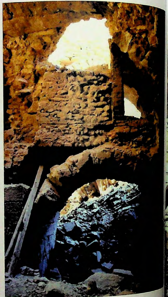
Figure 4.64. The higher rounded arch on the outside that may have once been composed of two levels of cross vaults.
