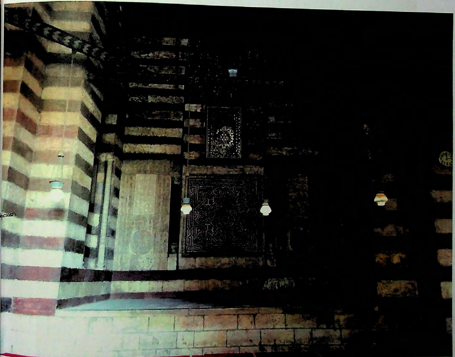
Figure 4.51. The mastaba in the vestibule of the Complex of Sultan Hasan.
