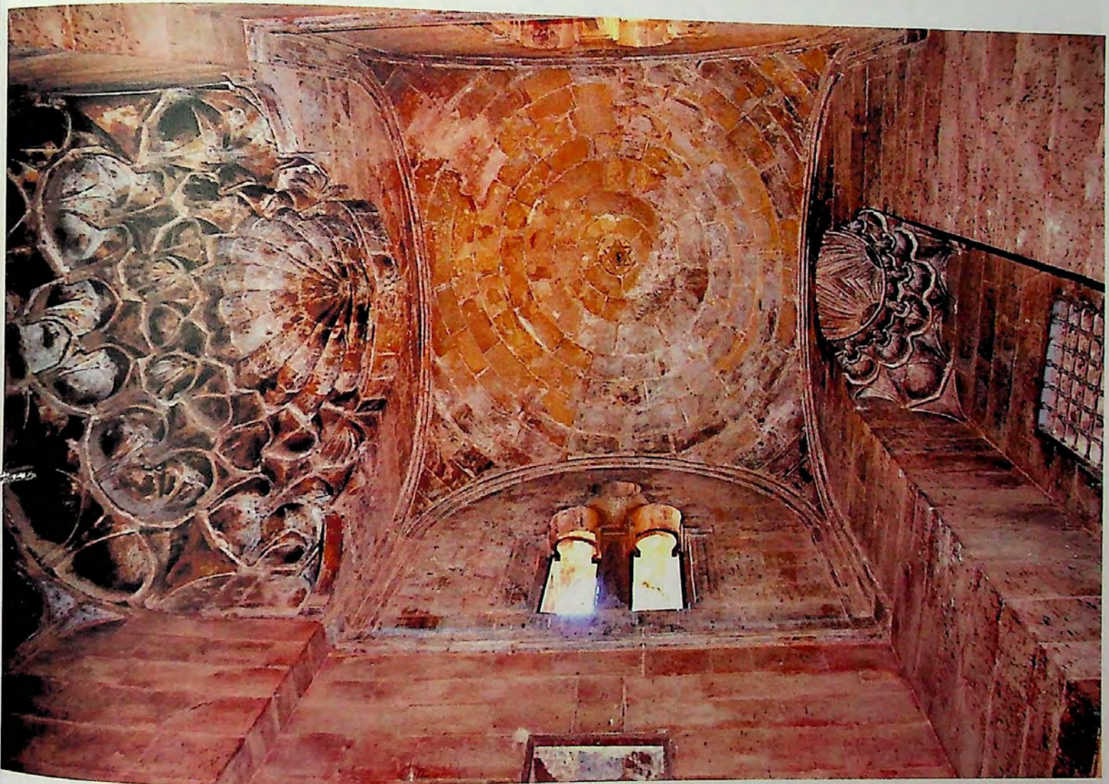
Figure 4.45. The vestibule of the palace.
