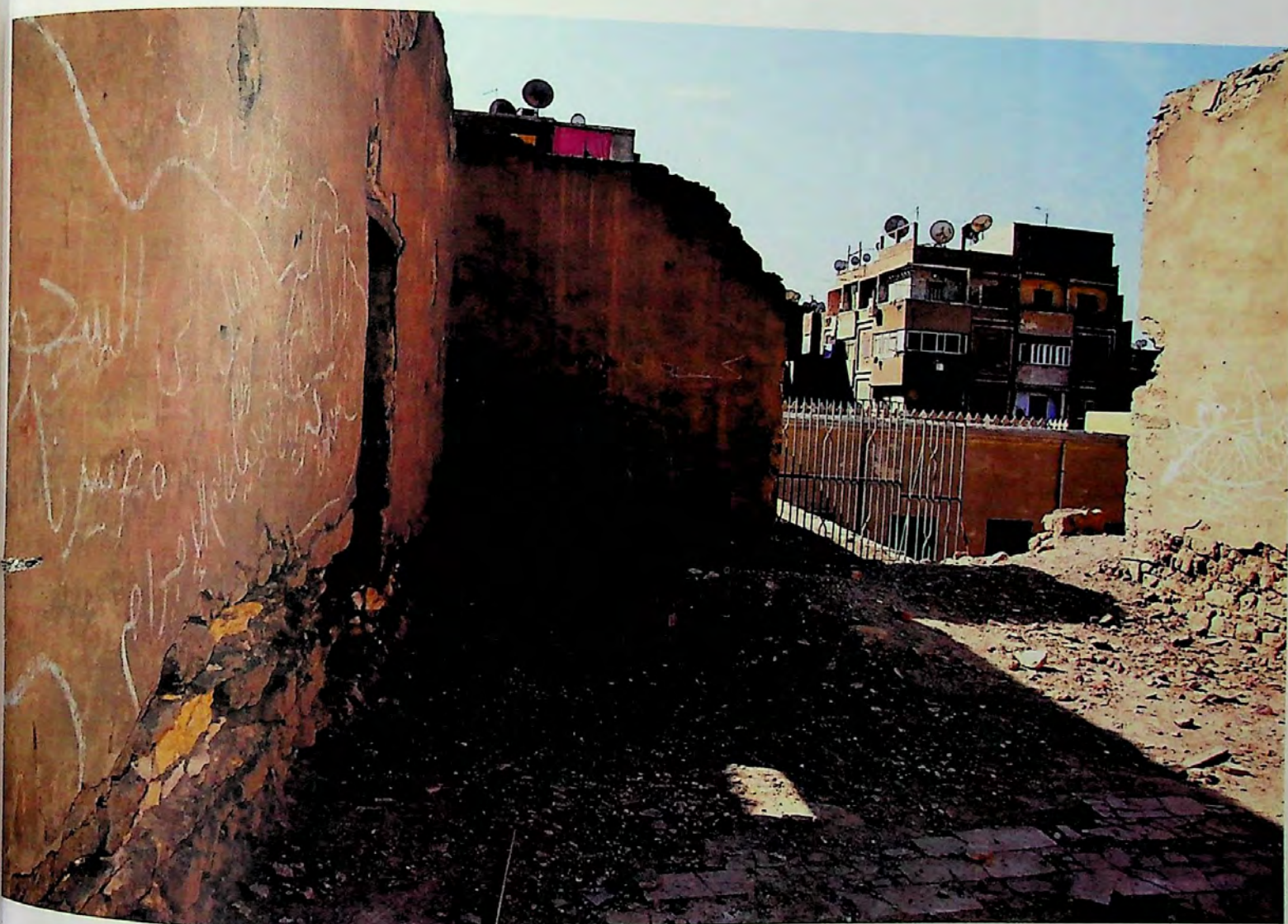
Figure 4.83. The qa'a (no. 21 on Plan G) with a number of rooms arranged around it.
