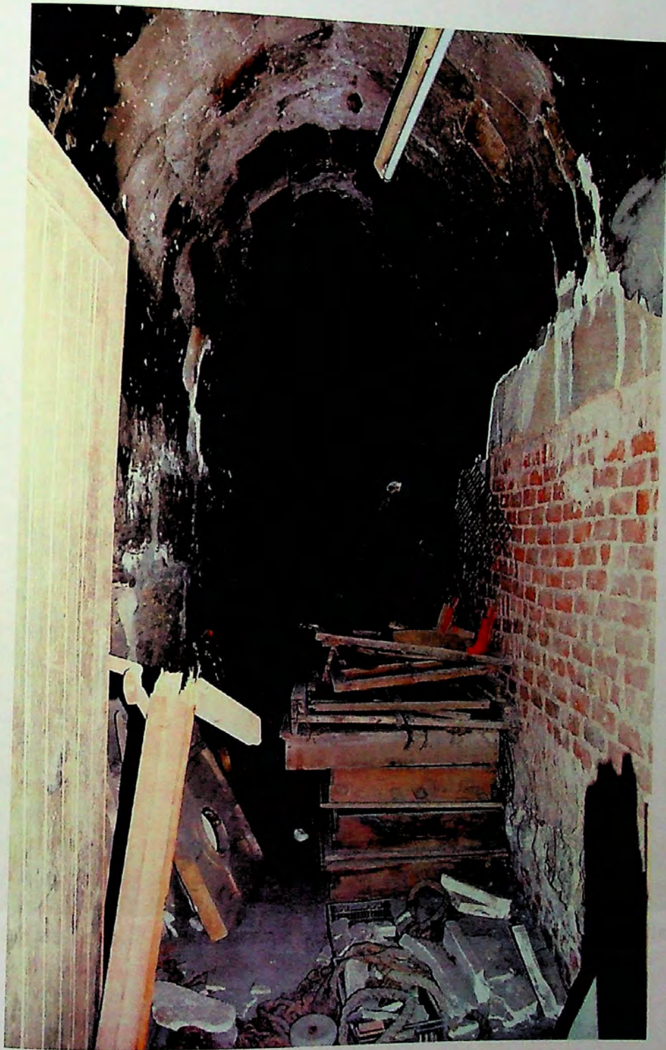
Figure 4.87. The corridor that once connected to the antechamber.
