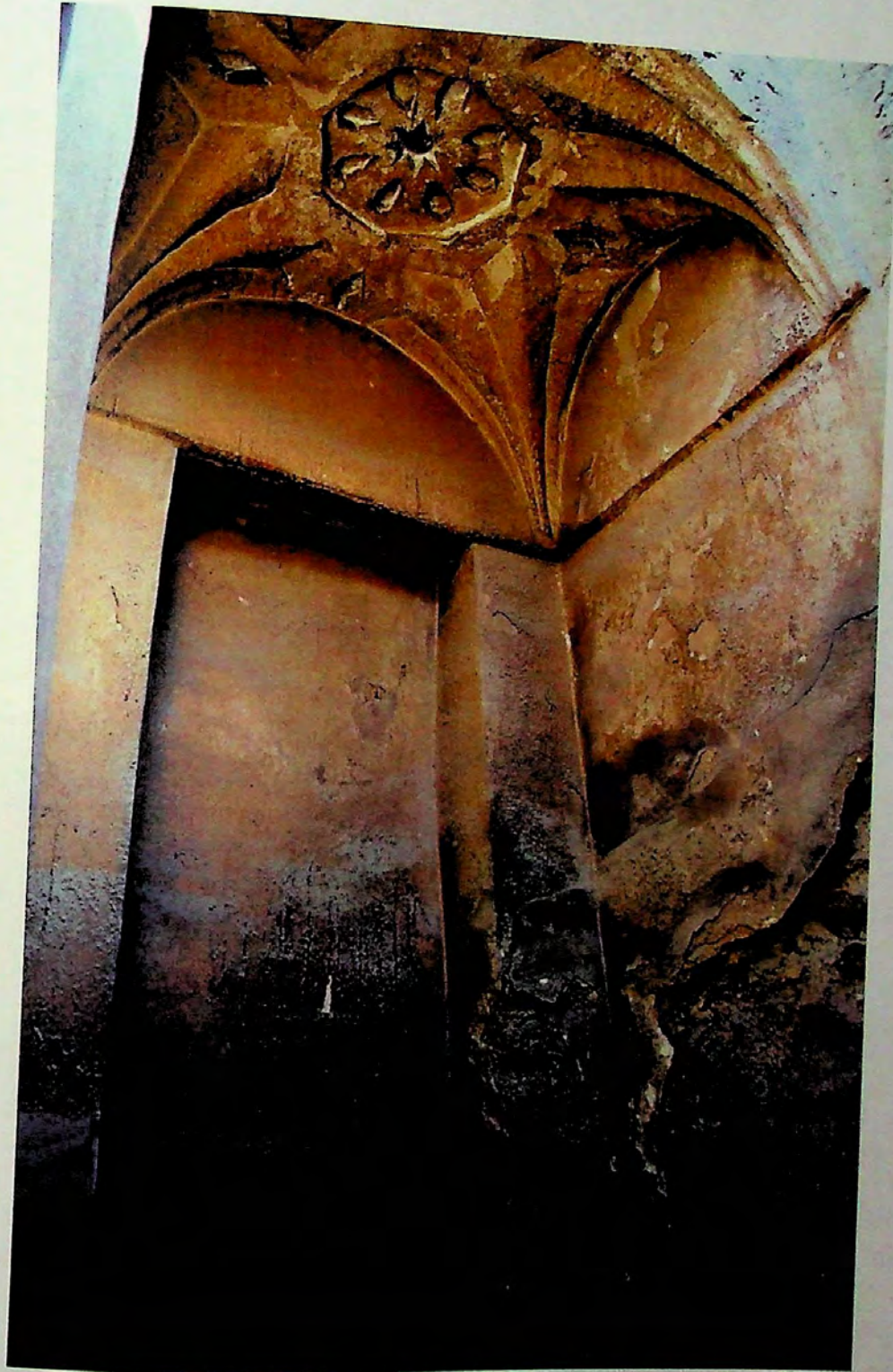
Figure 4.81. A latrine topped with a groin vault decorated with a geometric star ornament.
