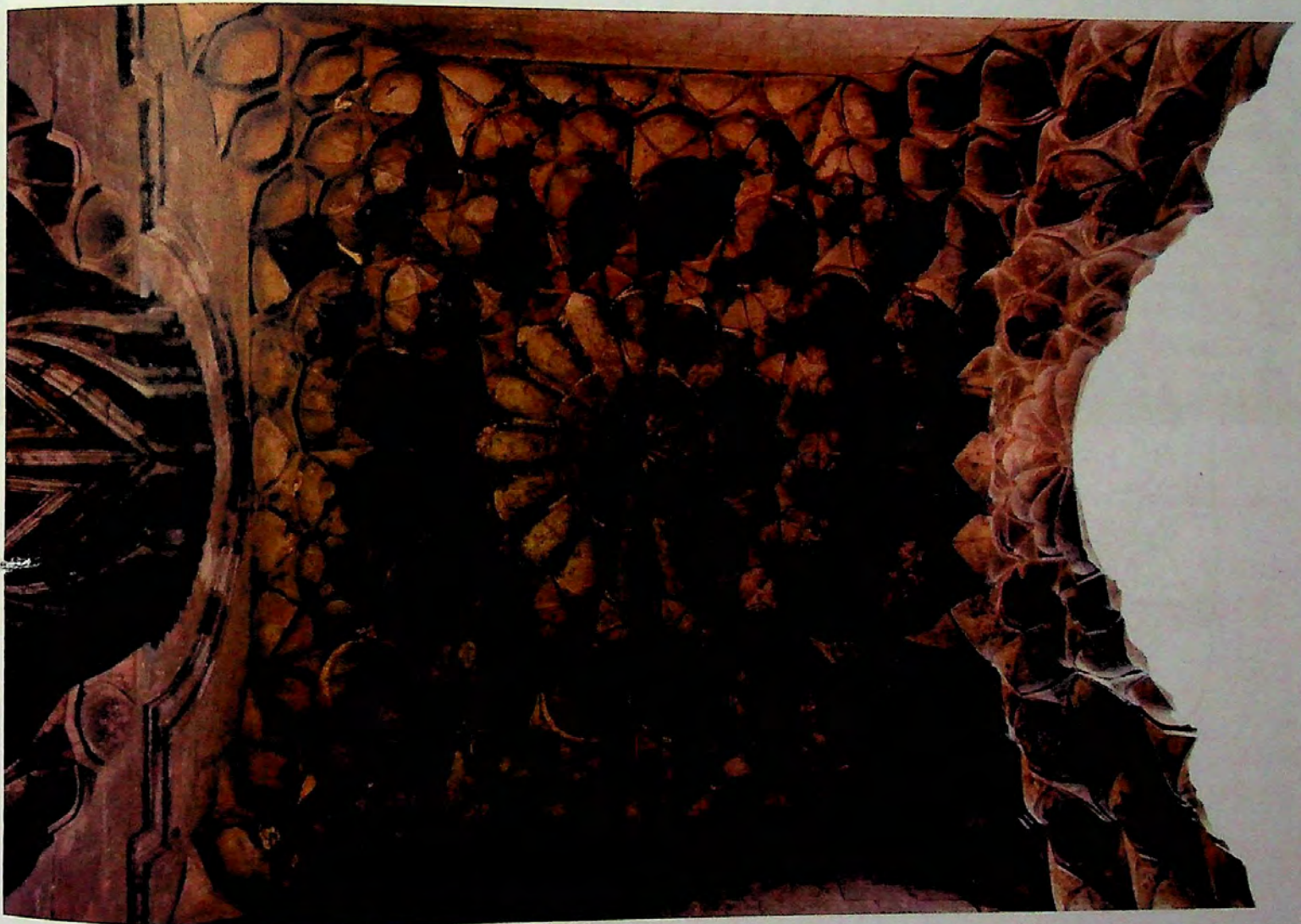
Figure 4.19. Detail of the muqarnas canopy of the portal of the Palace of Qawsun.
