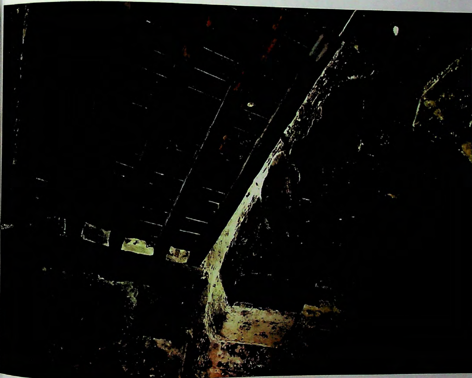
Figure 4.55. The central arch beam that supports the 'room of the guard' on the left.
