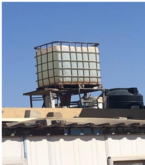
Figure 2.13: AUC WWT: Step 2: Chlorine Disinfection Tank
