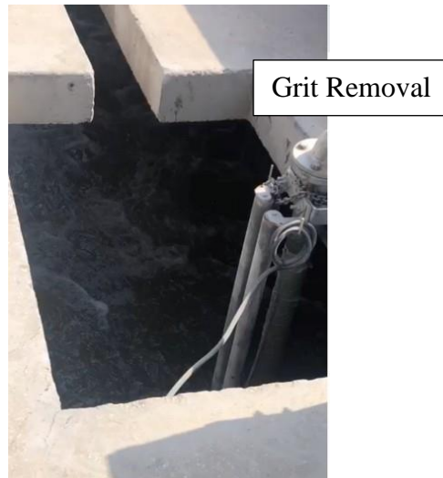
Figure 2.16: Madinaty WWT: Step 2: Grit Removal
