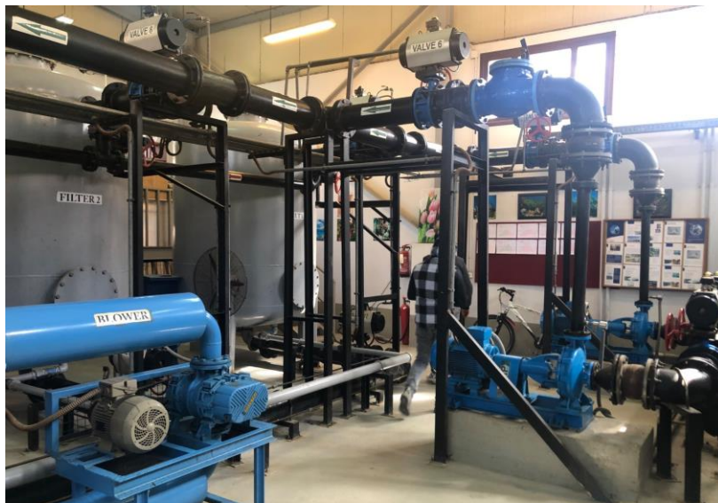
Figure 2.11: AUC WWT: Piping and Pumps connection with the Sand Filters for WWT delivery
