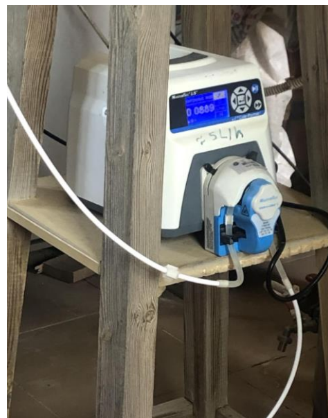
Figure 4.6: Pump between the Sedimentation Tank and the Sand Filters
