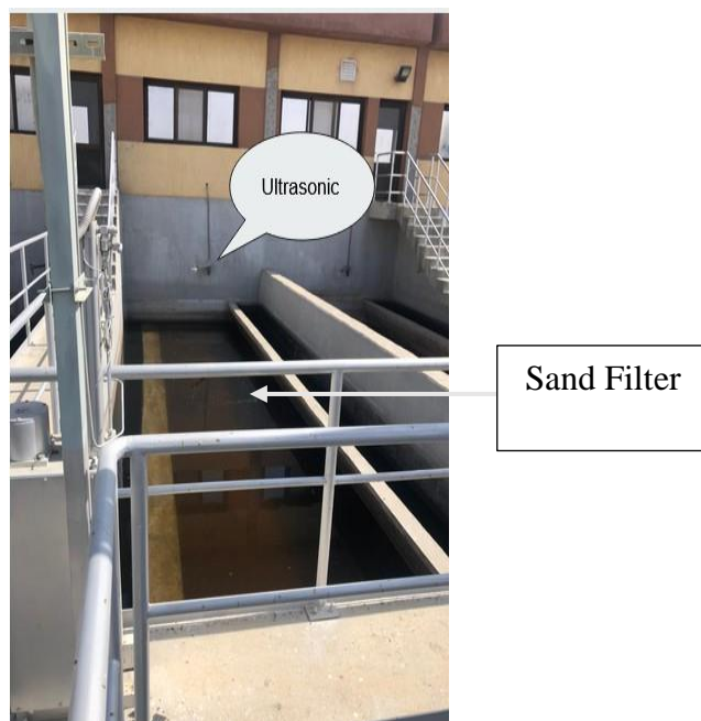
Figure 2.18: Madinaty WWT: Step 4: Sand Filter
