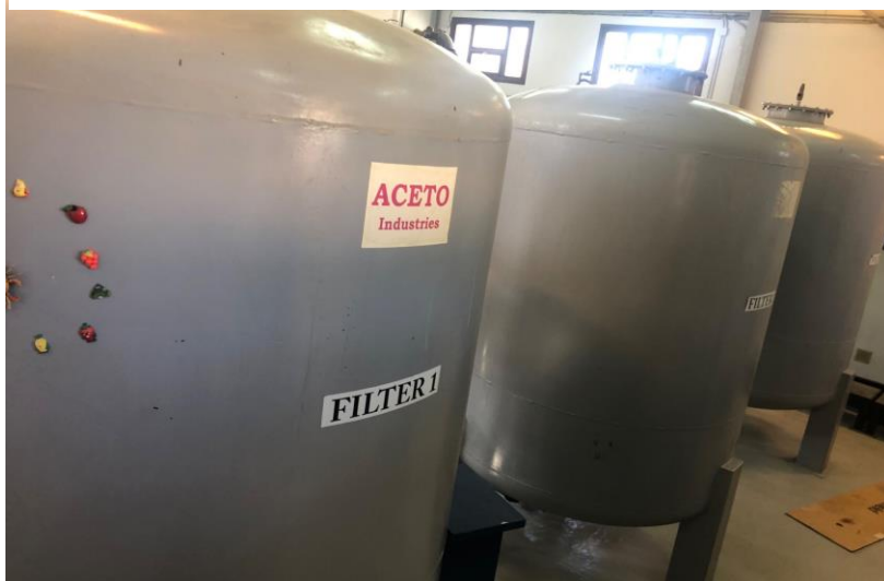
Figure 2.12: AUC WWT: Step 1: Sand Filters
