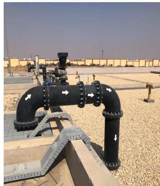
Figure 2.19: Madinaty WWT: Step 5: Chlorination
