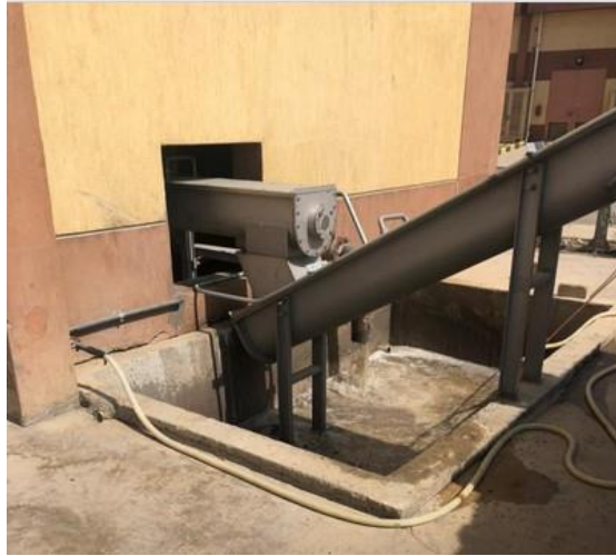
Figure 2.20: Madinaty Sludge Treatment: Step3 - Sludge Compression, Wastewater Out
