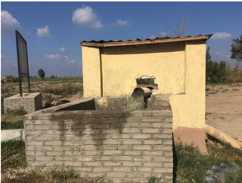
Figure 11: 23 meters deep well source
