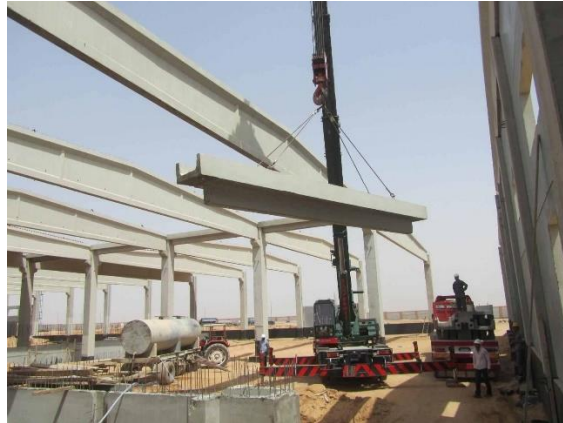
Figure 3.6: Image of rafter beams fixation on site. Drainage raft beam being moved by crane
