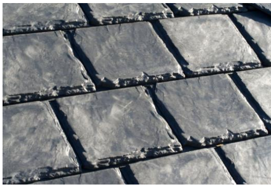
Figure 2.10: Recycled tires used in shingles (Green material, 2013)
