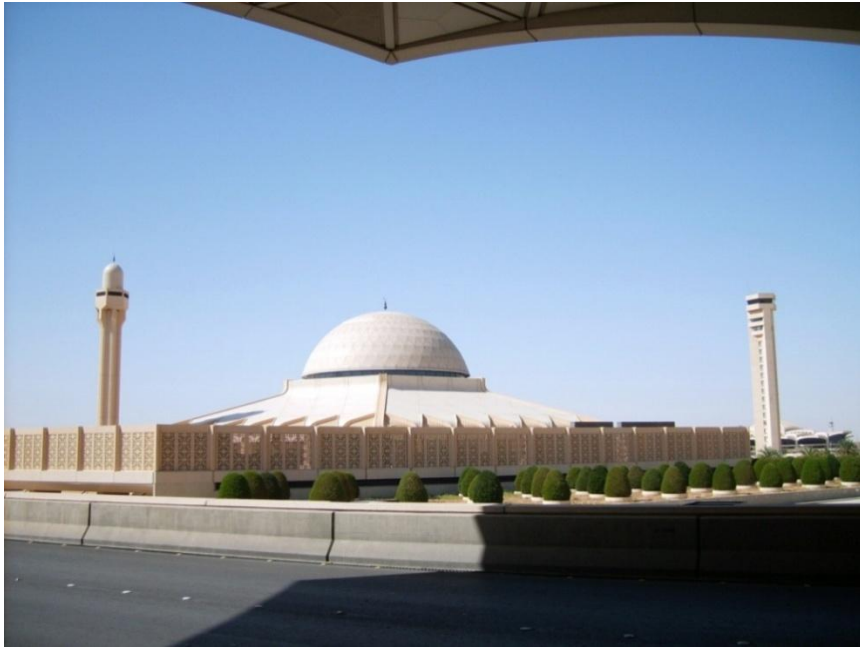
Fig. 29 King Khalid International Airport Mosque (Riyadh, 1983).
