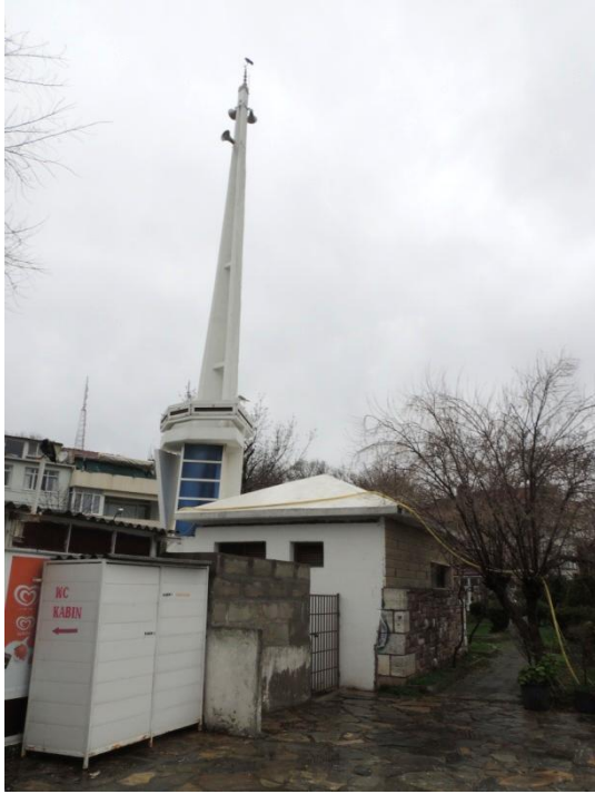
Fig. 31 Kinali Island Mosque, East Façade.
