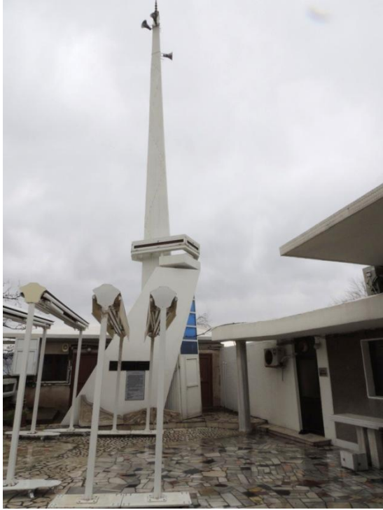
Fig. 39 Kinali Island Mosque, view of the minaret
