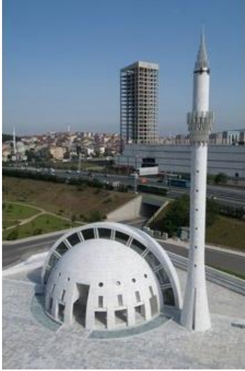
Fig. 132 Yeşilvadi Mosque, north façade with entrance.
