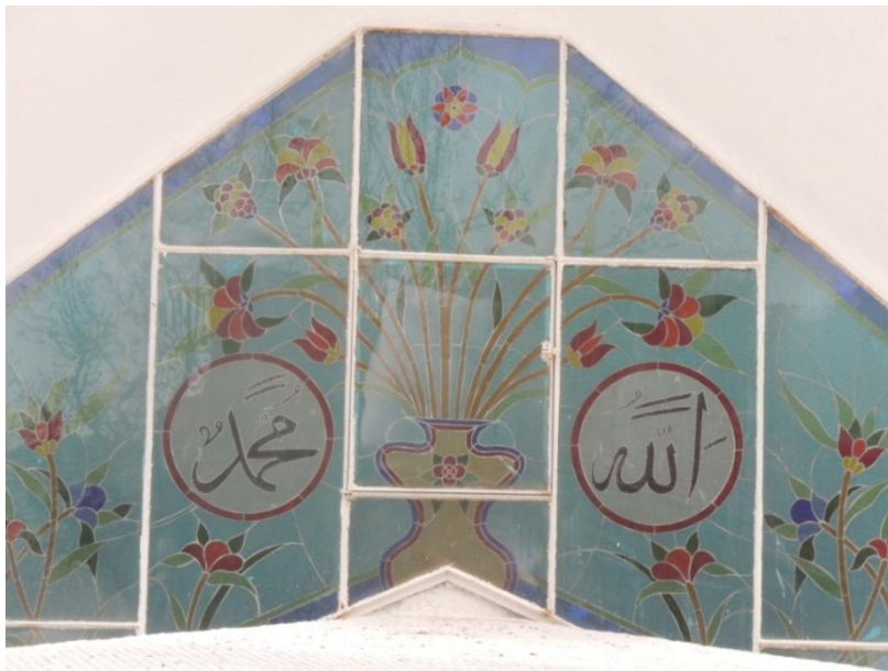
Fig. 42 Kinali Island Mosque, roof details from exterior
