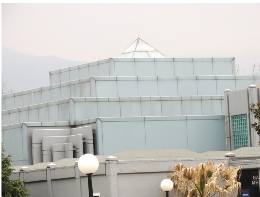
Fig. 119 Buttim Mosque, roof details of main prayer hall.
