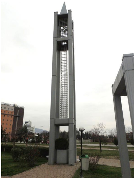
Fig. 121 Buttim Mosque, view of the minaret.
