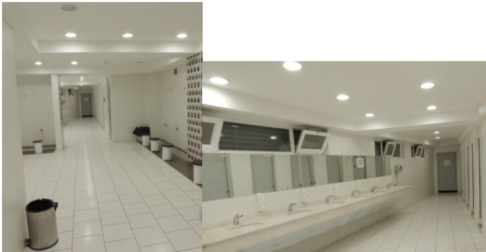
Fig. 172 Şakirin Mosque, women's restroom and ablution facilities
