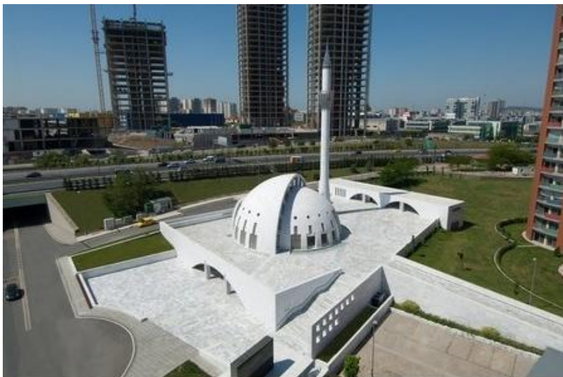
Fig. 131 Yeşilvadi Mosque, general view of the mosque and the piazza.
