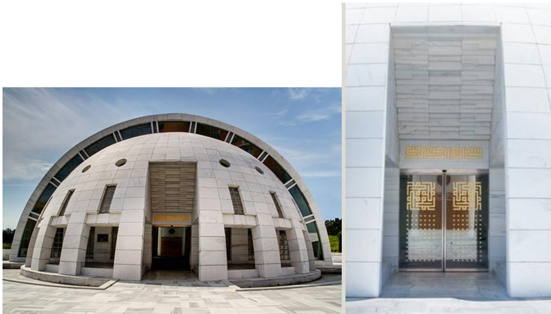
Fig. 135 Yeşilvadi Mosque, main entrance to prayer hall and sliding door.
