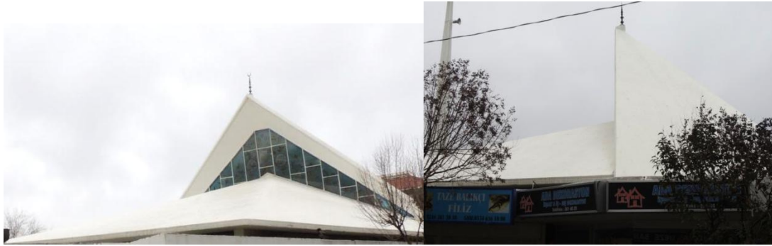
Fig. 41 Kinali Island Mosque, frontal and side view of the roof
