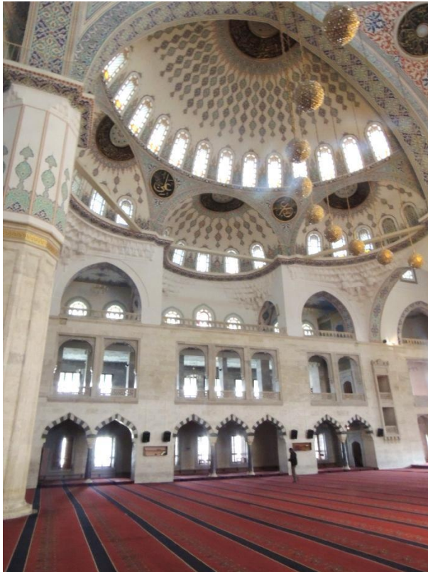
Fig. 65 Kocatepe Mosque, interior of the prayer hall with view of side surrounding galleries.
