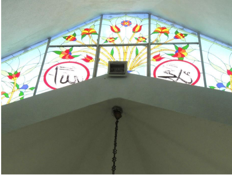
Fig. 43 Kinali Island Mosque, roof details from interior
