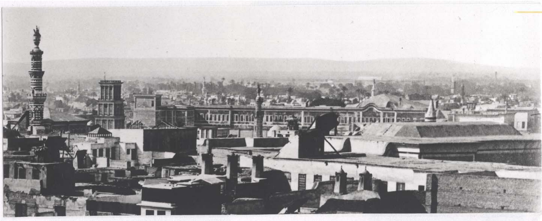
Pl. 4.11 Nineteenth century photograph of Saray al-Hilmiyya, after Tamraz (watchtower is very prominent in this photograph)
