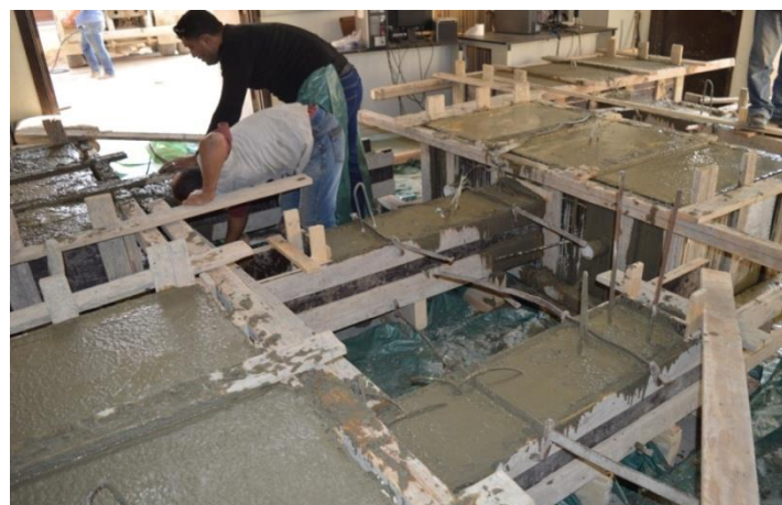
Figure4.30: Checking the leveling during pouring concrete
