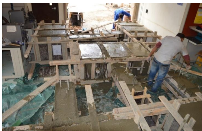
Figure 4.34: Final check after pouring
