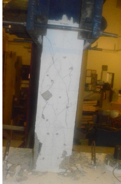
Figure 5.102: CSS-15-E Crushing concrete cover of 3.72\Delta y
