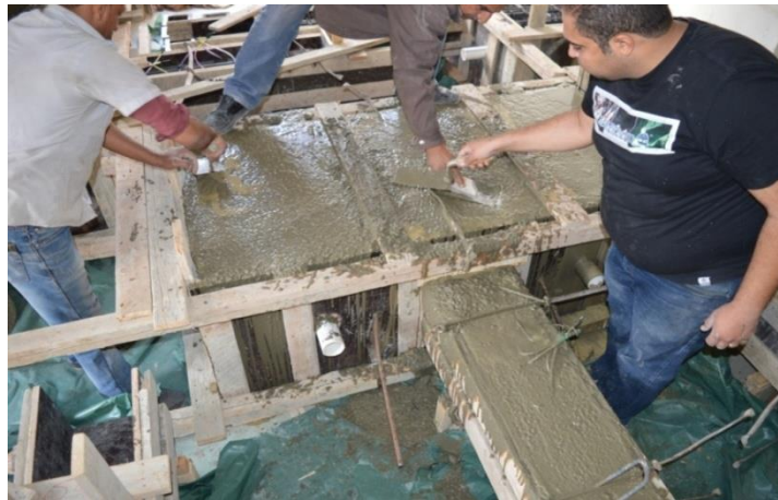
Figure 4.32: Finishing the pouring face of concrete
