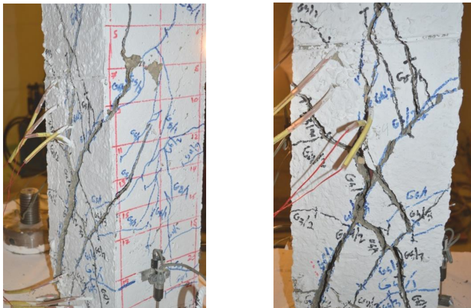
Figure 5.135: CSS 40-E Opening cracks 2.856 \Delta y
