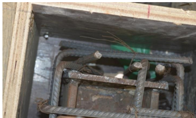
Figure 4.27: The column head
