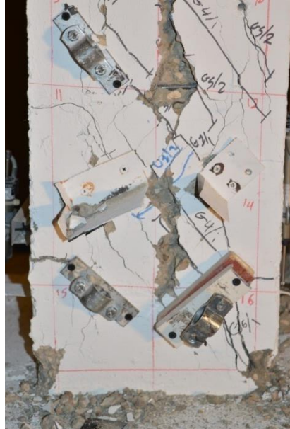
Figure 5.117: CSS-20-ECrushing concrete cover mid cycle of (2.85 \Delta y )
