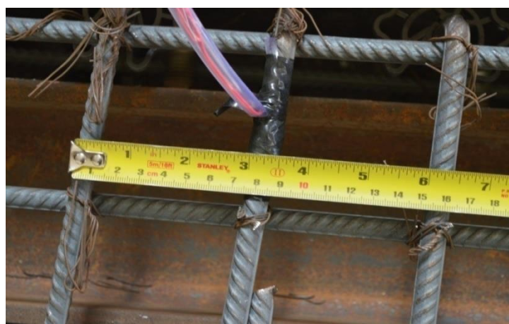
Figure 4.25: Checking the stirrups spacing
