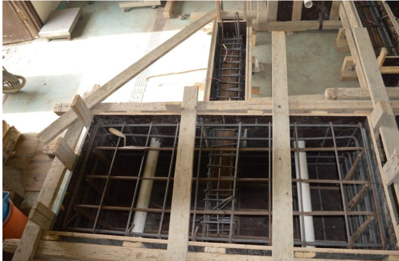
Figure 4.21: Plywood fair face form work
