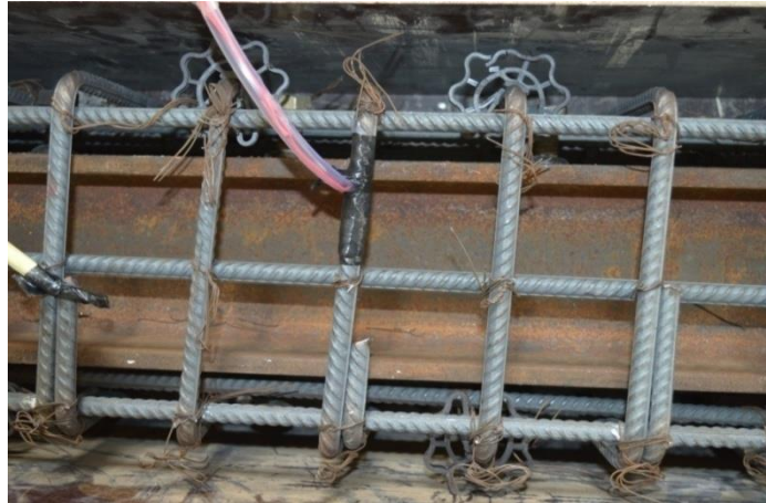
Figure 4.26: Checking the accuracy of concrete cover
