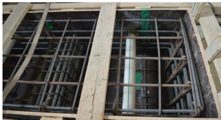
Figure 4.24: Making the groves for the tubes of the fixation bolts
