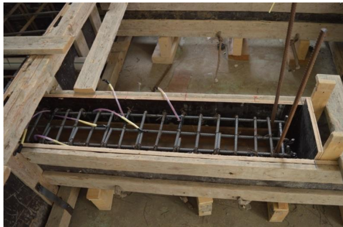
Figure 4.22: Leveling of specimen column
