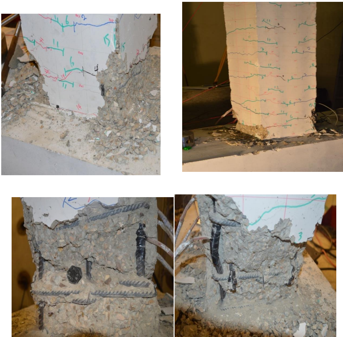
Figure 5.2: Failure mode of specimen CSF10-NP
