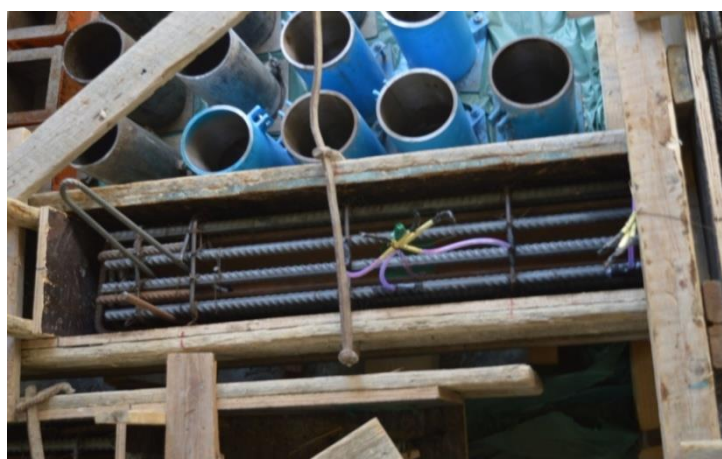
Figure 4.28: Fixing the strain gages as designed
