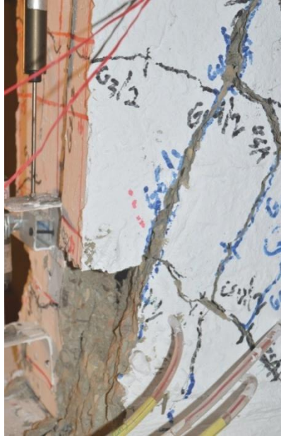
Figure 5.136: CSS 40-ECrushing concrete cover ( 3.71 \Delta y )
