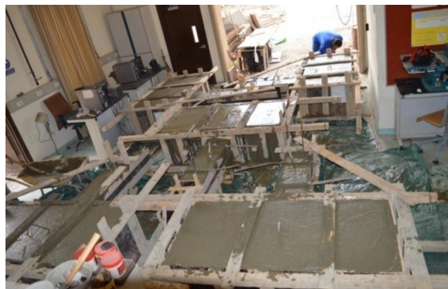
Figure 4.33: Pouring all specimens
