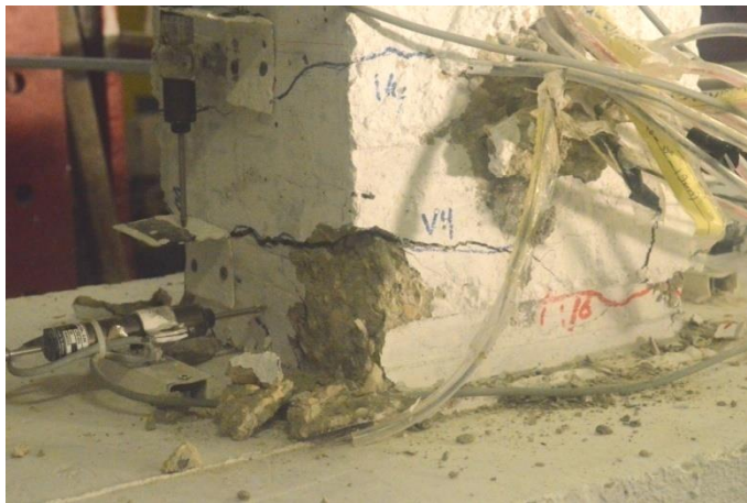
Figure 5.44: CSF-10-75 Crushing concrete cover mid cycle of (2.197 \Delta y )
