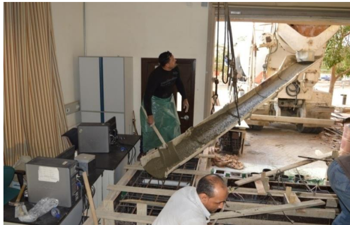
Figure 4.29: Pouring with ready mix concrete
