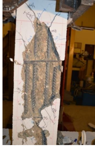
Figure 5.119: Final failure of column CSS-20-Econcrete cover ( 3.71\Delta y )
