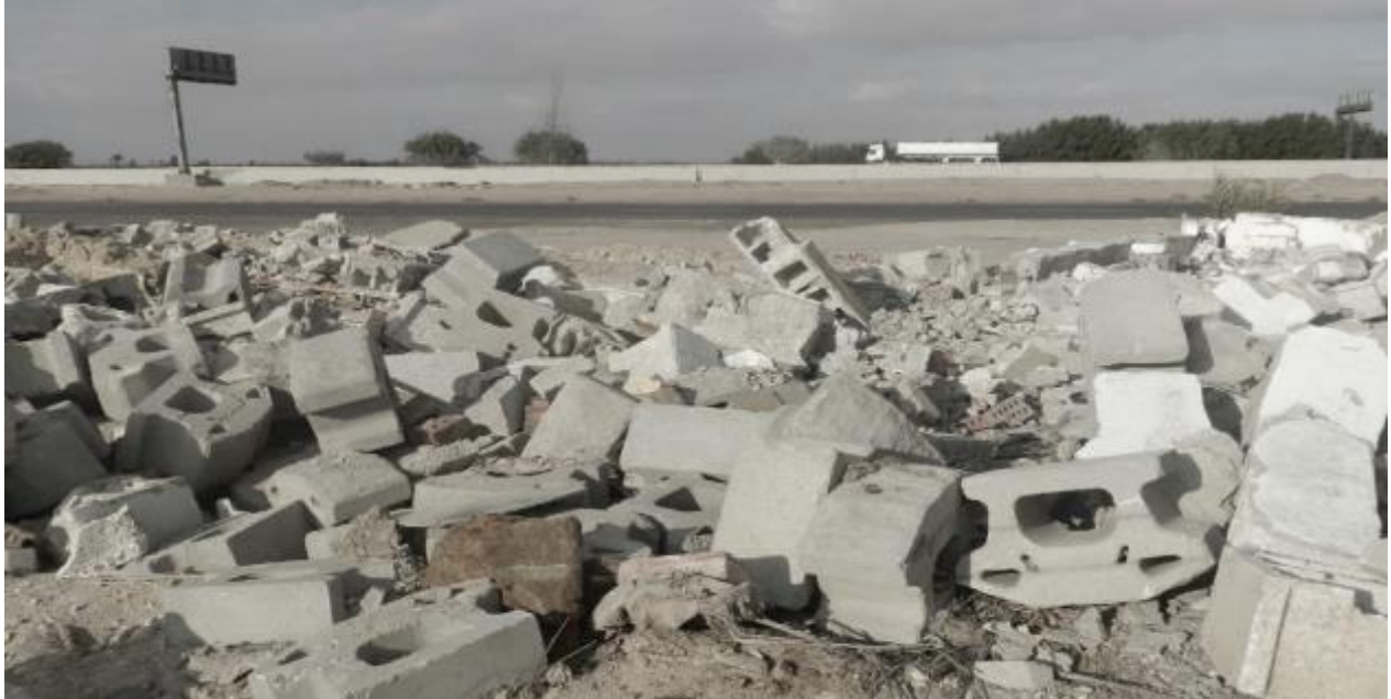
Figure 1.1 The ruins of a demolished shop, Ard Baza, 2016 (Photographed by author).
