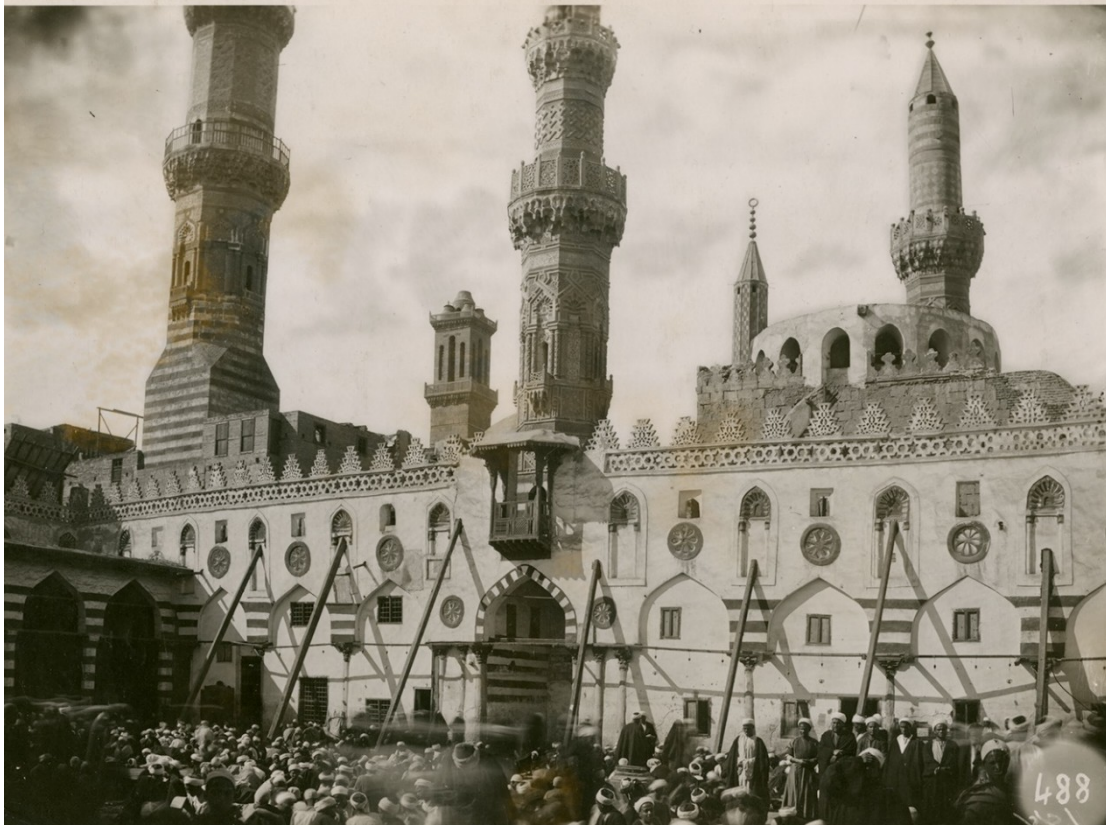
Figure 44: A photograph showing the northwestern façade of al-Azhar mosque during the restoration by the Comité (photo before the 10 th century from the personal collection of Sir Creswell). Courtesy of the Rare Books and Special Collections Library.
