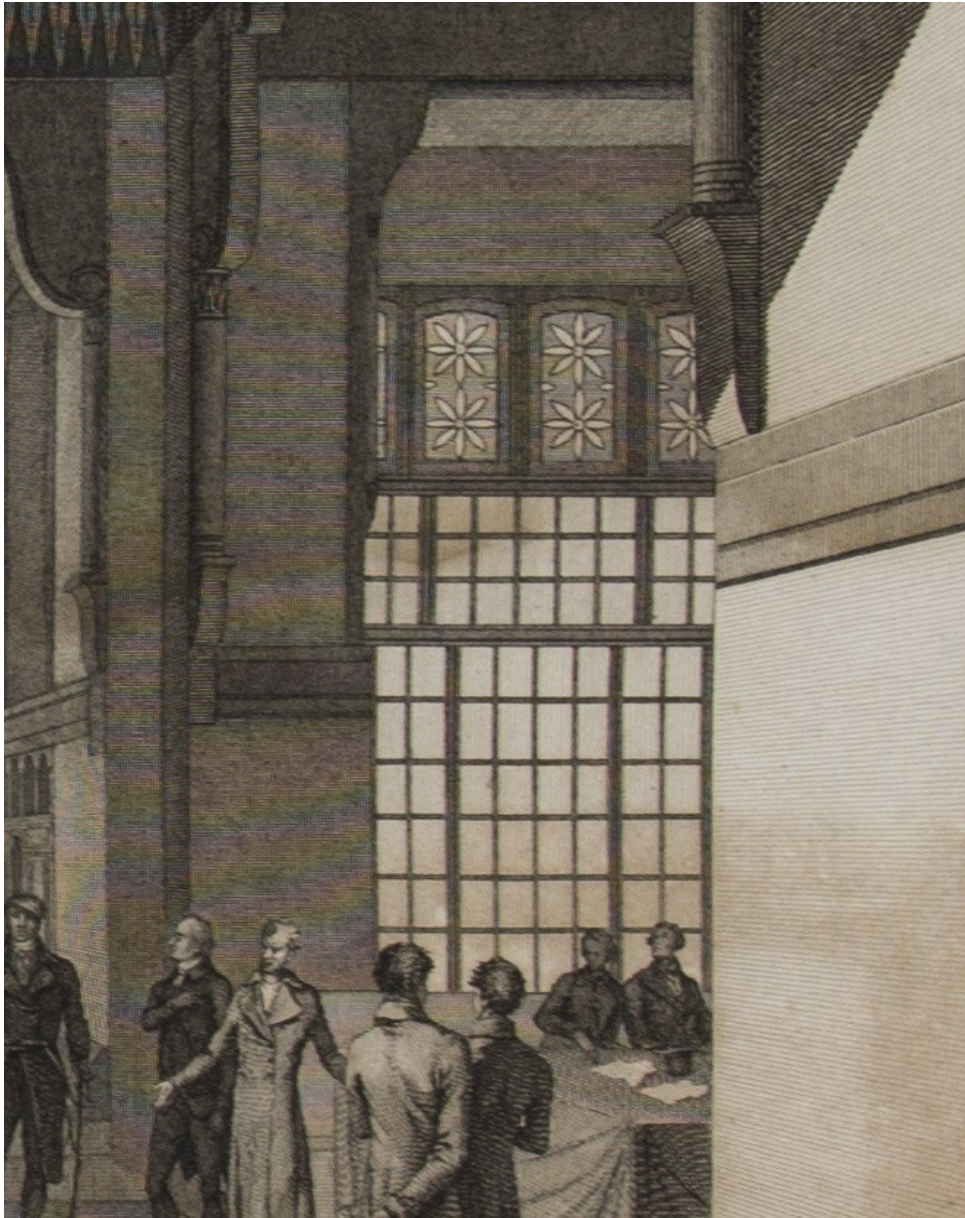
Figure 118: Detail of the mashrabiyya and the colored-glass windows (lithograph before 1809) (after La description de l’Egypte, état moderne , vol. 1). Courtesy of the Rare Books and Special Collections Library, the American University in Cairo.
