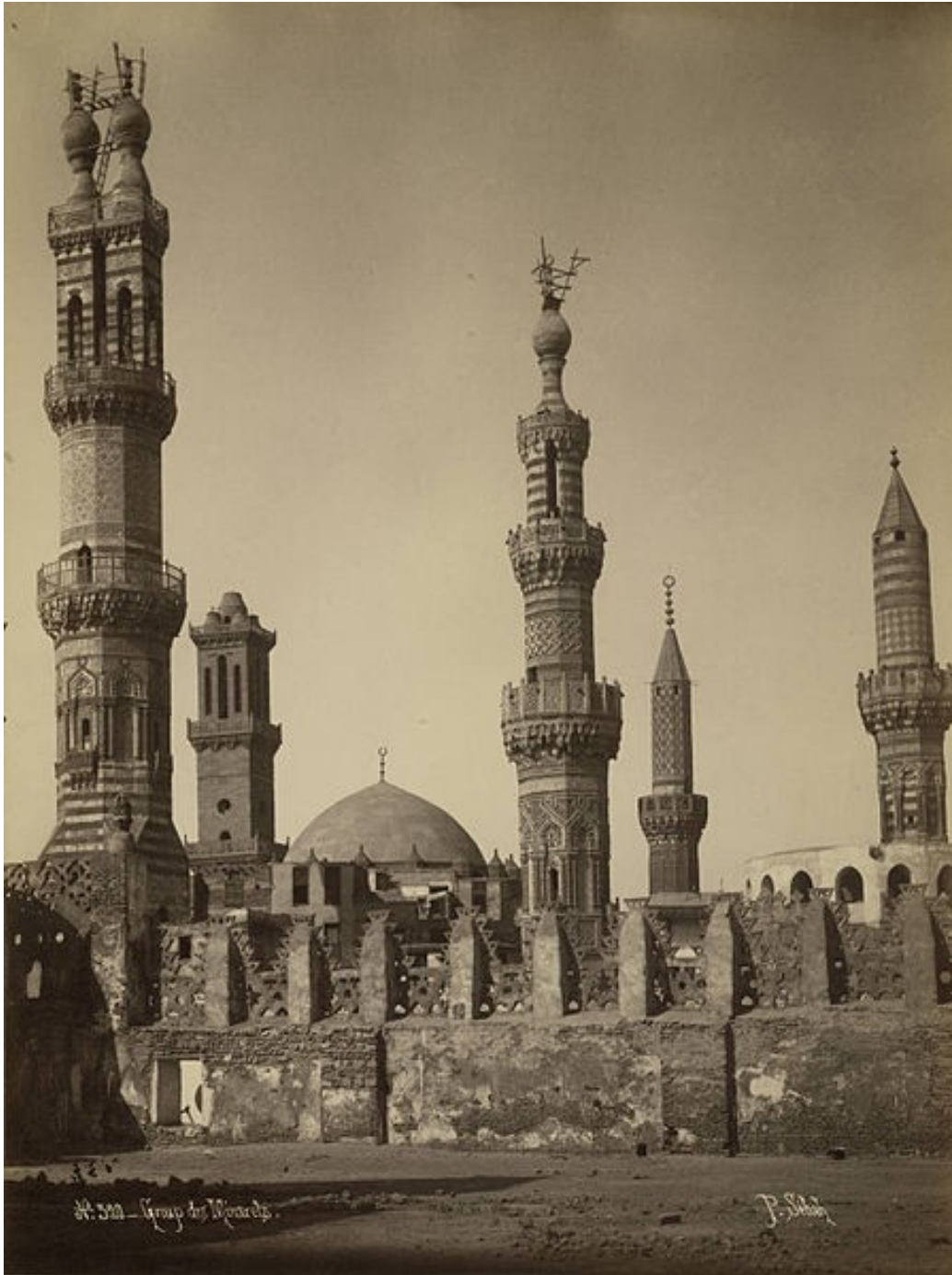
Figure 43: The northwestern façade of the al-Azhar mosque, the group of minarets and the non-extant dome of the Aqbughawiyya madrasa (photo before 1887 by Pascal Sebah) (after Wikimedia Commons, accessed from https://commons.wikimedia.org/wiki/File:Egypt._Group_of_Minarets.jpg ).
