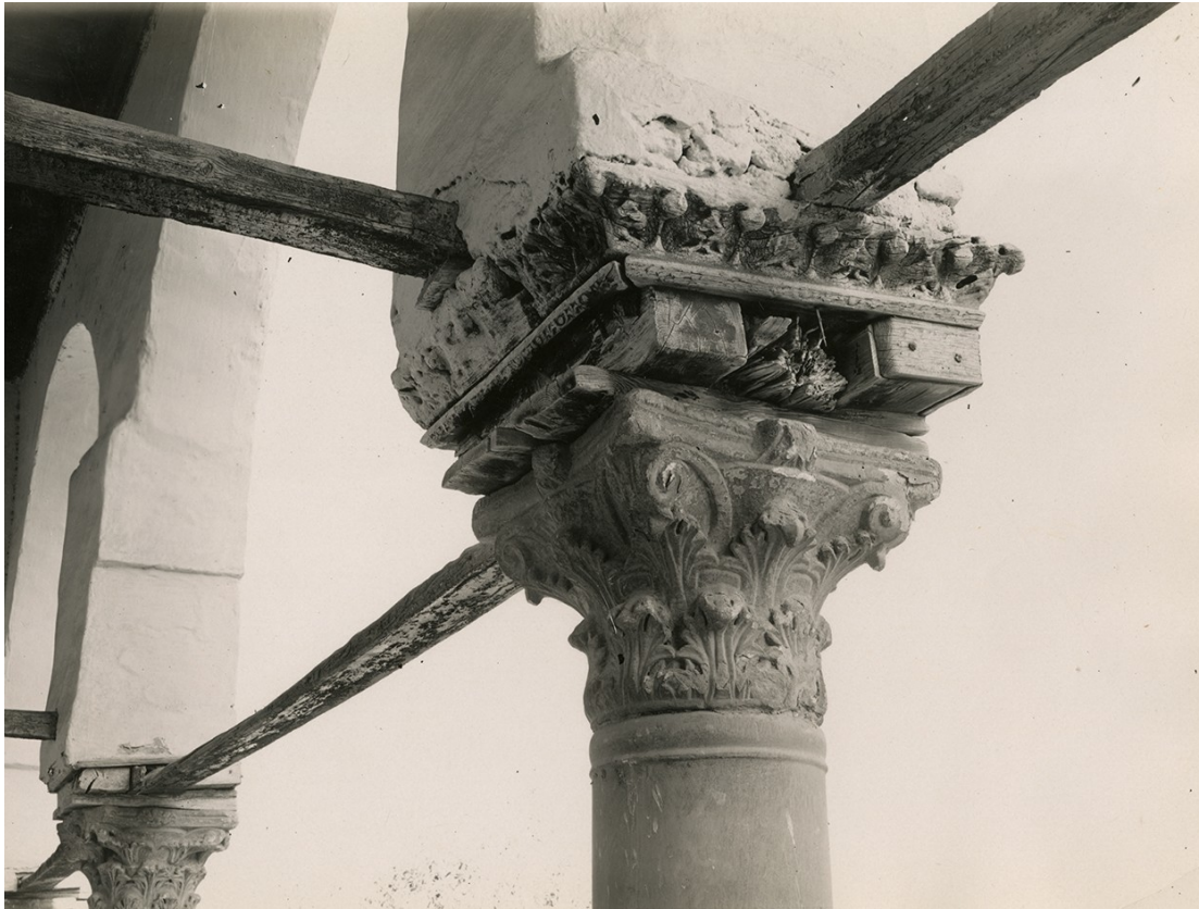
Figure 88: A photograph showing the detail of the Corinthian capitals and the wooden beams in the sanctuary of the mosque of 'Amr (photo from the personal collection of Creswell before the 20 th century). Courtesy of the Rare Books and the Special Collections Library, the American University in Cairo.
