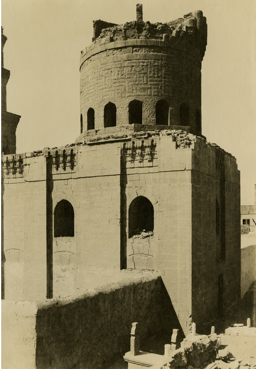
Figure 33: A photograph showing the dome of the Sultaniyya mausoleum collapsed (photograph from the personal collection of Creswell before the 20 th century). Courtesy of the Rare Books and Special Collections Library.
