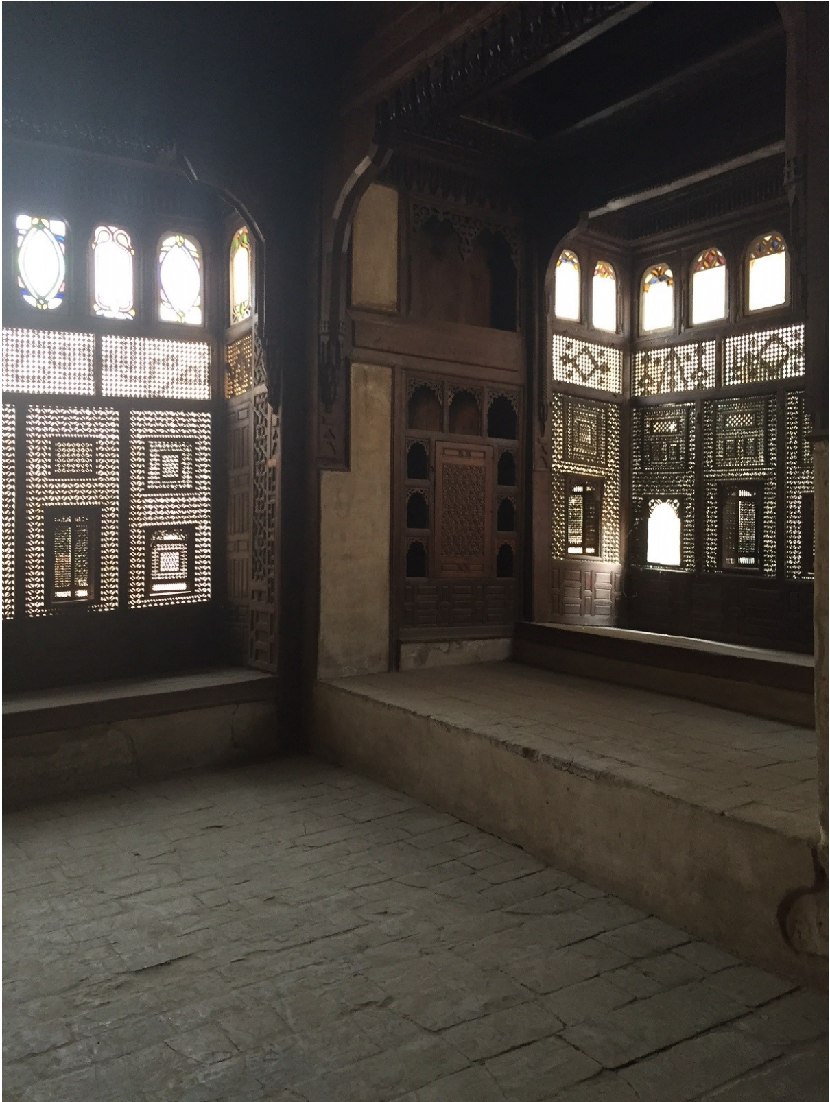
Figure 123: The conserved mashrabiyyas, the color-glass windows, the wooden built-in cupboards and the pavement (photo before 2017 by Heba Sheta).
