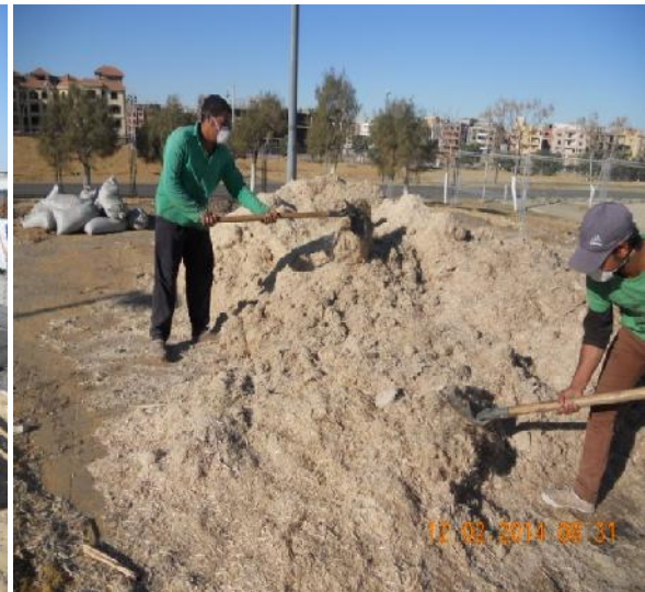
Figure 3.15. Preparing compost windrows
